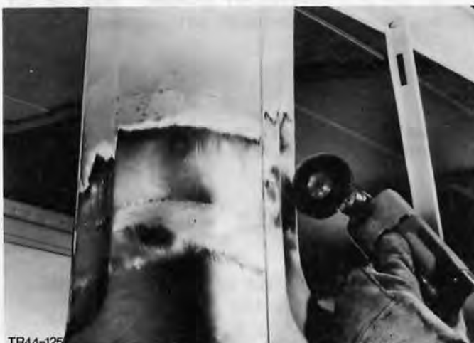
Fig.188. Dress joint seam.
